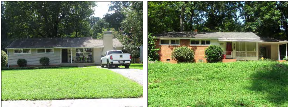
Figure 37: L to R, an example of a house that has lost its integrity of design due to a filled-in garage at one end at 2515 Overbrook Drive and an example with an integrated carport at 2518 Westmoreland Drive.
