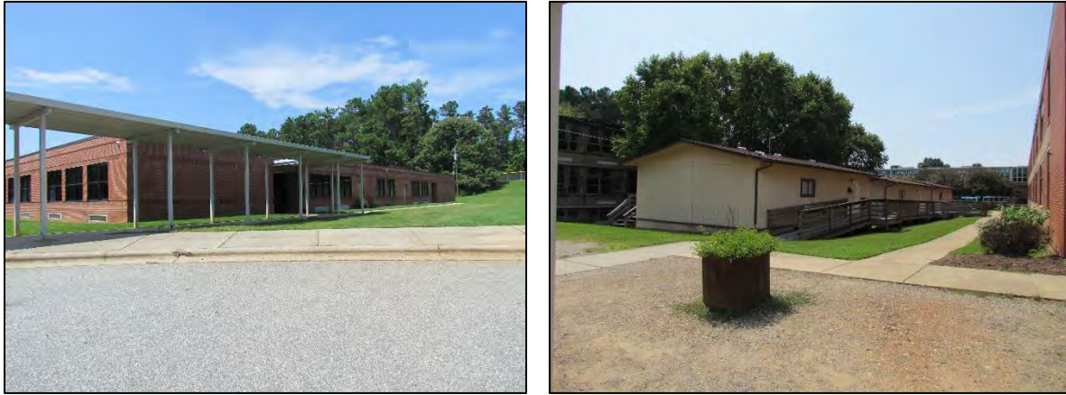
Figure 26: L to R, covered walkway leading to Building 9 and the courtyard between Buildings 3 and 4, with the east elevation of Building 2 visible in the background.
