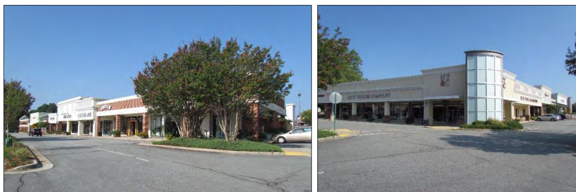
Figure 11: Building A, left, and Building C, right.
