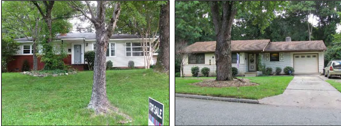
Figure 36: L to R, a Transitional Ranch with two types of siding, hipped roof, and Modernist corner window at 1104 Quail Drive and an example with two siding types, a side-gable roof, and an attached garage at 1201 Surry Drive.
