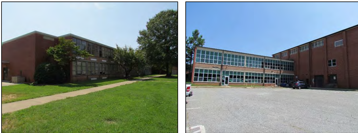
Figure 25: L to R, the north elevation of Building 3 showing part of courtyard and a view of Buildings 5 and 6.
