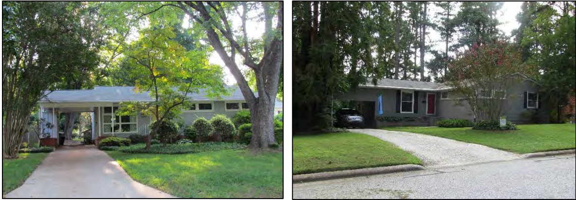
Figure 42: L to R, Two Modernist one-story homes with integrated carports at 1406 Quail Drive and 2501 Westmoreland Drive.
