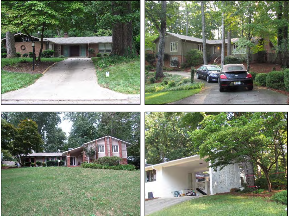
Figure 67: Clockwise from upper left, 1303 McDowell Drive is a single-story house with a prominent cross-gable, wide eaves, exposed beams, and triangular fixed paned clerestory windows flanking the roof ridge beam. It also has a single car garage integrated into gable and a decorative concrete screen obscures access to a side entrance. 1502 Ilchester Drive is L-shaped with low pitched gabled roofs. 1701 Swannanoa Drive features decorative concrete elements at the carport and at a patio wall. The rest of the home was obscured by heavy vegetation. 3305 Northampton Drive is a Split-Level house with simplified brick pilasters, a low pitched gabled roof with an elongated end that forms an entry porch.
