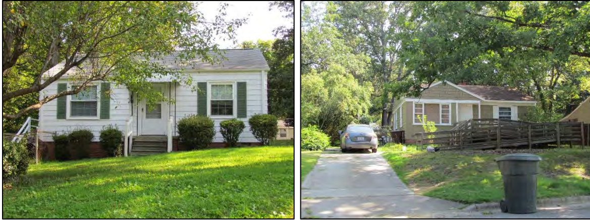
Figure 49: L to R: 2706 Shady Lawn Drive, an intact example of the Minimal Traditional and situated diagonal to an intersection; 2814 Shady Lawn Drive with diminished integrity due to the construction of a large wheelchair ramp.
